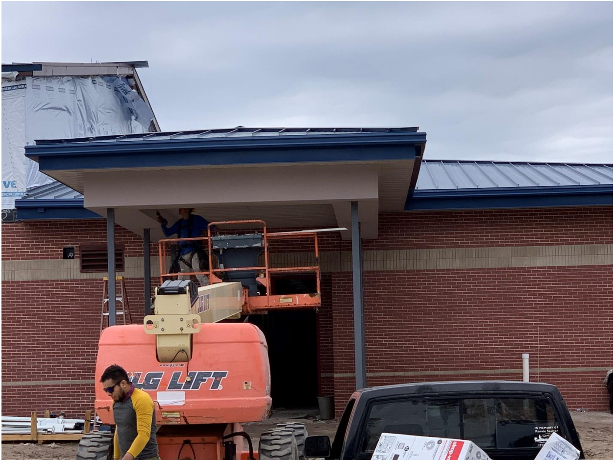
I was there just in time to take a picture of the last piece going into place.
